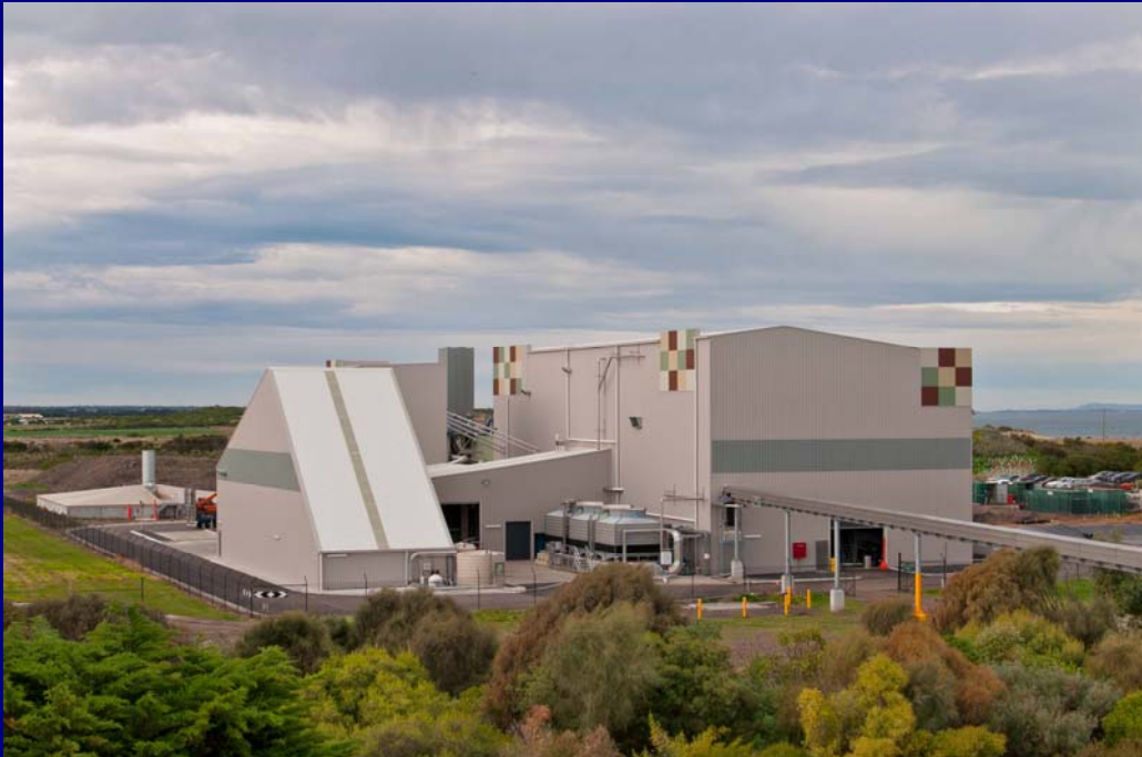
Rear view of the Facility as it nears completion
