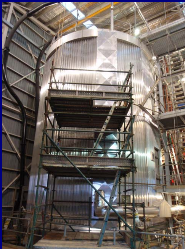
Construction and insulation of the dryers are substantially completed
