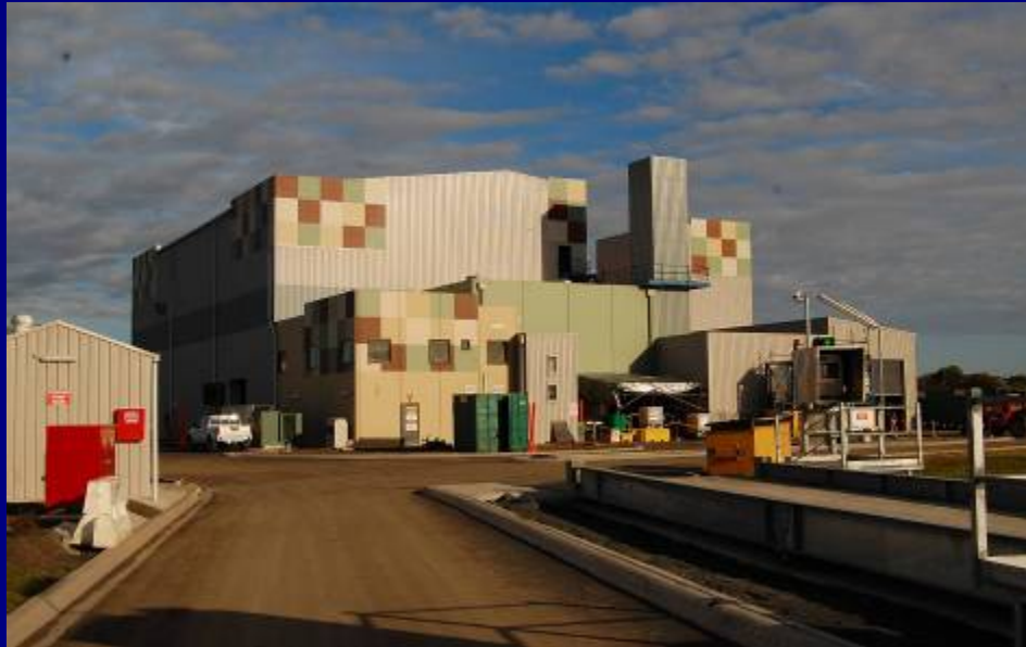
Front view of the Facility with the weighbridge to the right of the image
