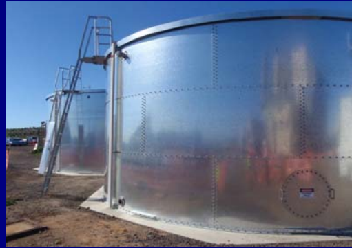
Installation of tanks.
