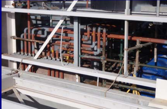
Process pipework and control valves are installed
