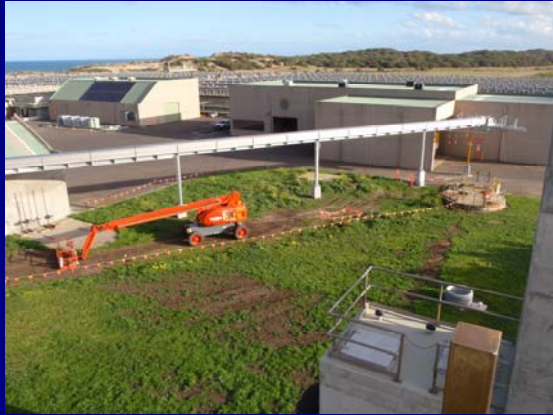
Installation fully enclosed conveyor is approaching completion
