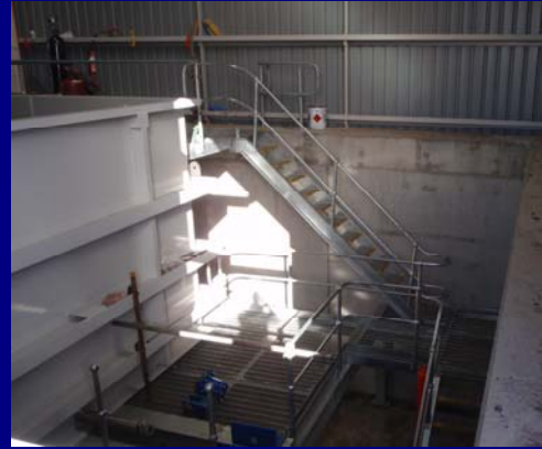
Installation of materials handling systems
