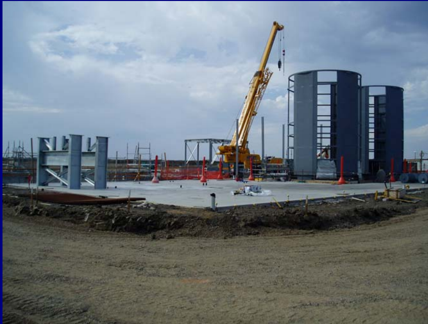
Installation of dryers and surrounding steel platforms and support structures.
