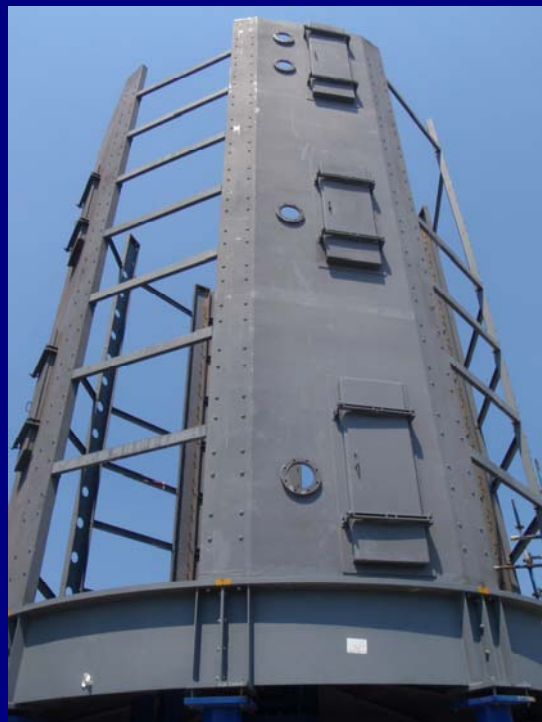
Construction of the dryer Keppel Seghers biosolids dryer shell.
