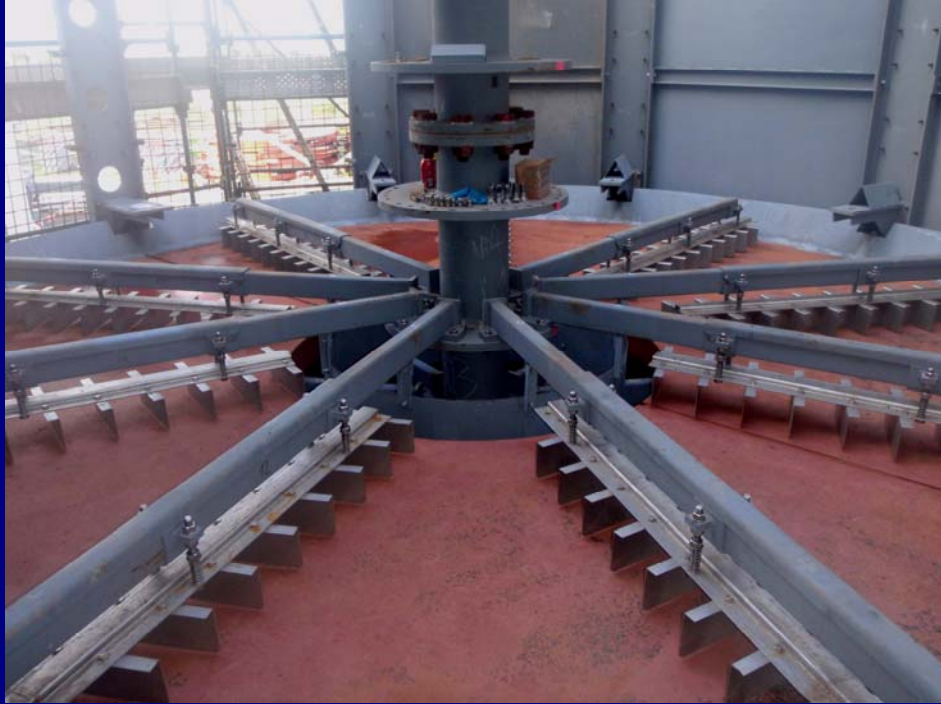
Installation of the dryer components.
