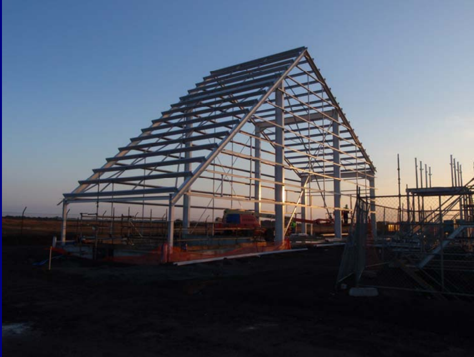
Steel framing of the imported biosolids building.
