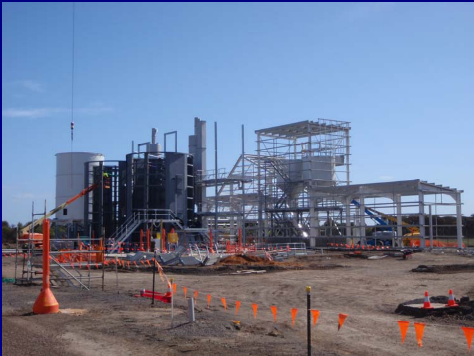
Installation of equipment and construction of building framework.
